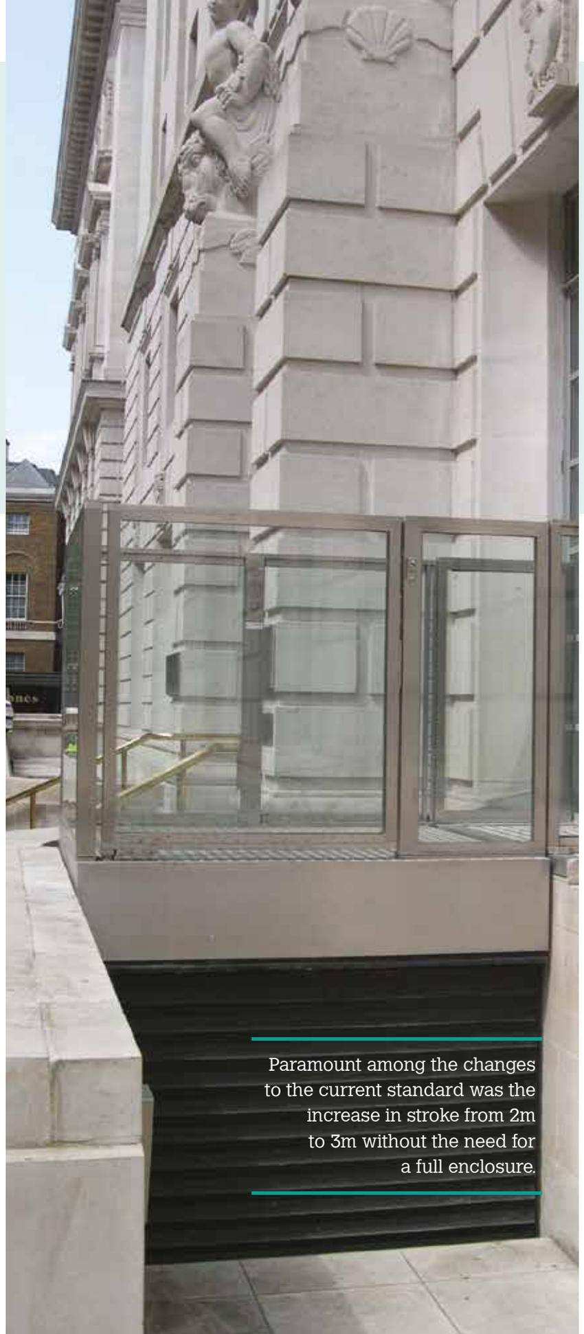
Paramount among the changes to the current standard was the increase in stroke from 2m to 3m without the need for a full enclosure.
